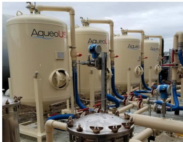
AV's scope included prefiltration, fabricated steel and PVC manifold piping, ion exchange vessels, sensors for controls monitoring, on-site installation, and system pressure testing.
