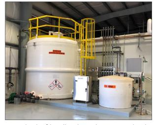
and operating costs, as well as the cost and risk of handling hazardous materials. The DOW compared bulk sodium hypochlorite, calcium hypochlorite and On-Site Sodium Hypochlorite Generation (OSHG). The result of their detailed evaluation pointed to the OSHG option as meeting their needs for safety, self-sufficiency, independence and resiliency while achieving the lowest life cycle costs for the DOW.
